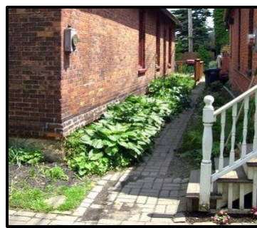
Path between buildings
